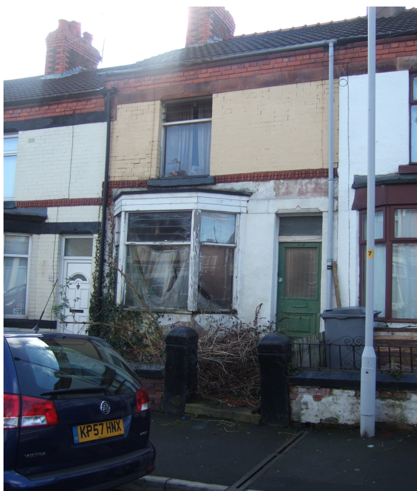
Figure 1 - Initial Inspection of Property
